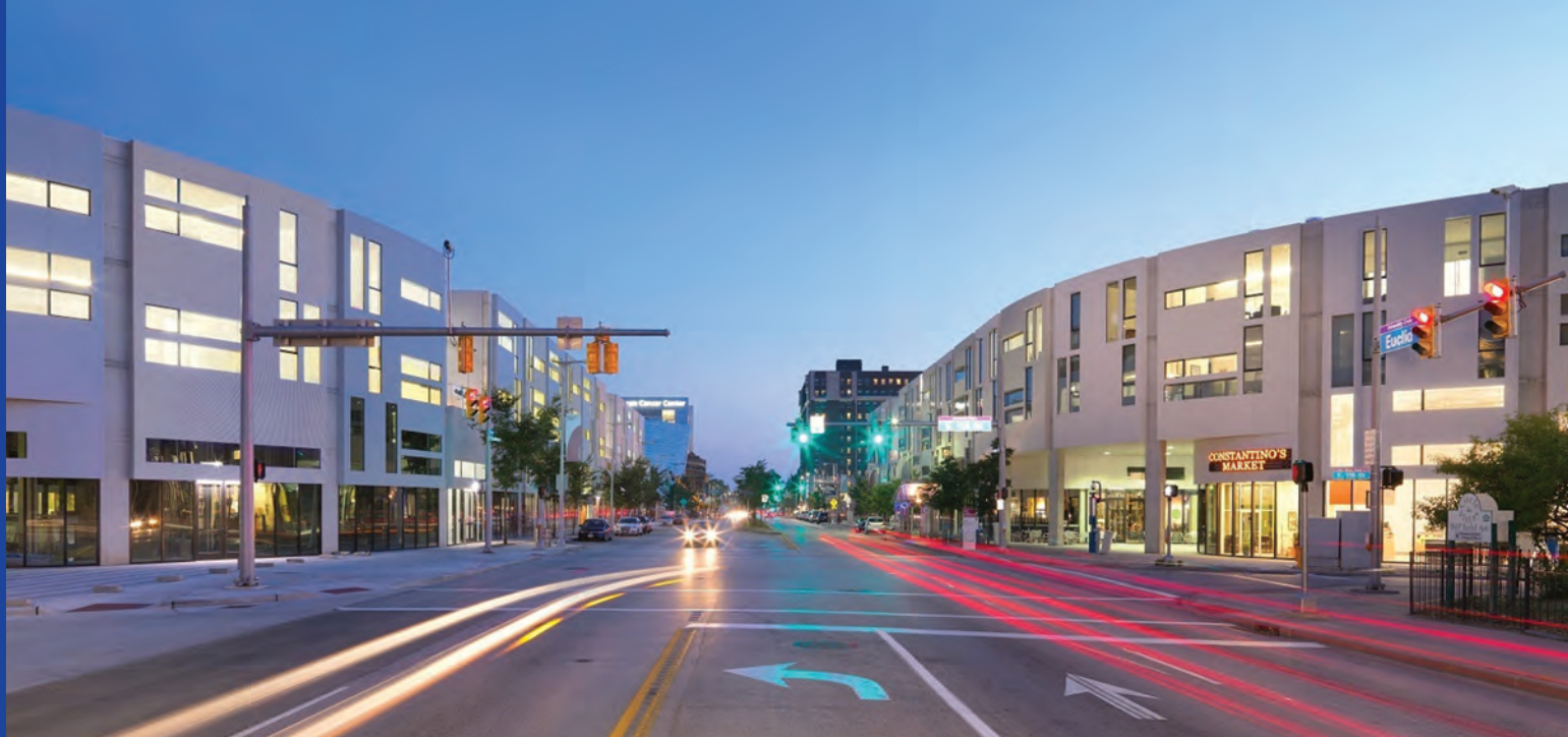
Uptown, the new mixed-use development in the University Circle area, is set to tie together the institutions of University Circle. Photo courtesy of KeyBank
